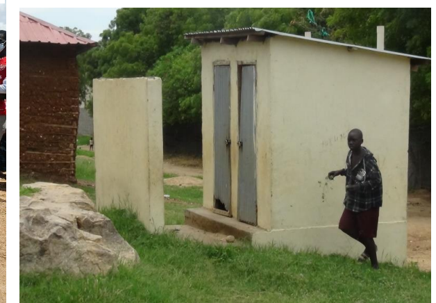
Yo' Care constructed sanitation facility in Tolmere Namere, Juba, CES, 2022.
